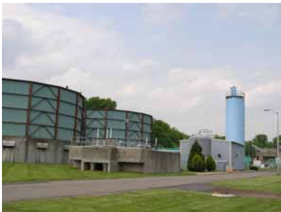
Quakertown Sewer Plant
