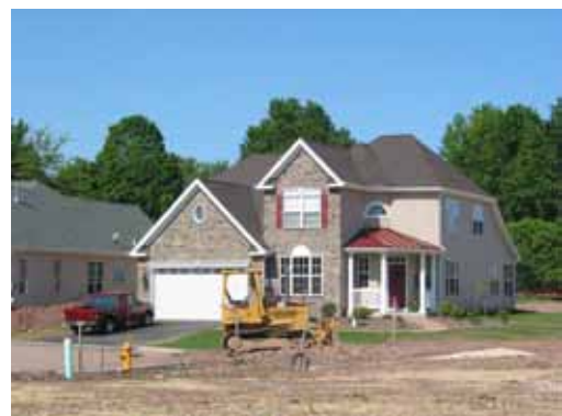
Renaissance age-restricted housing in Richland (under construction)
